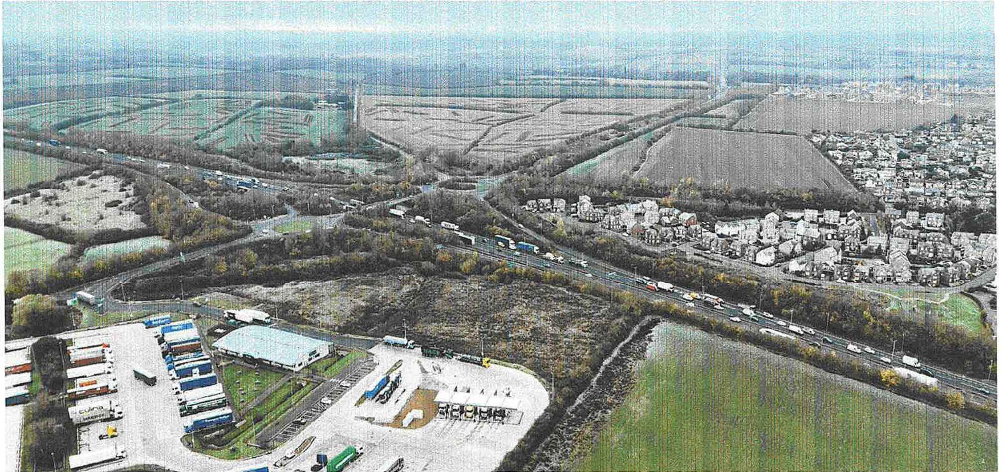
View looking south east with Rothwell to the west. Views of the site and buildings from Rothwell will be clearly seen
