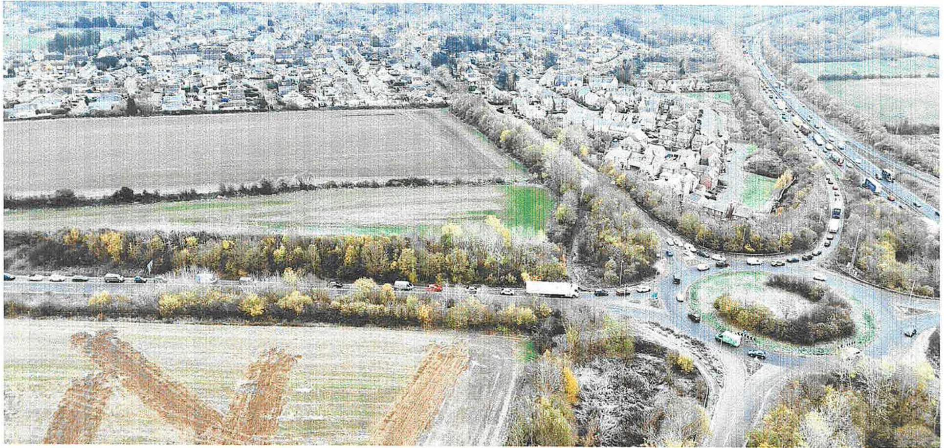
View looking north-west towards Rothwell from the corner of the site.
